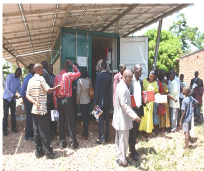
Participants inspect the solar container
