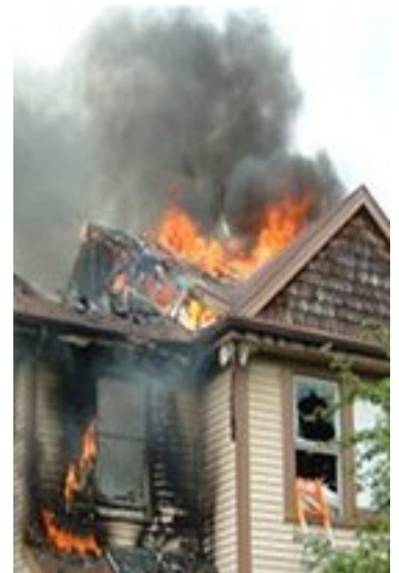
House fire caused by poor electrical installation.
